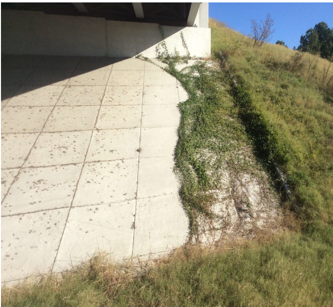
PHOTO 1 Description Abutment #1 concrete slope on left side has vines growing on it.
