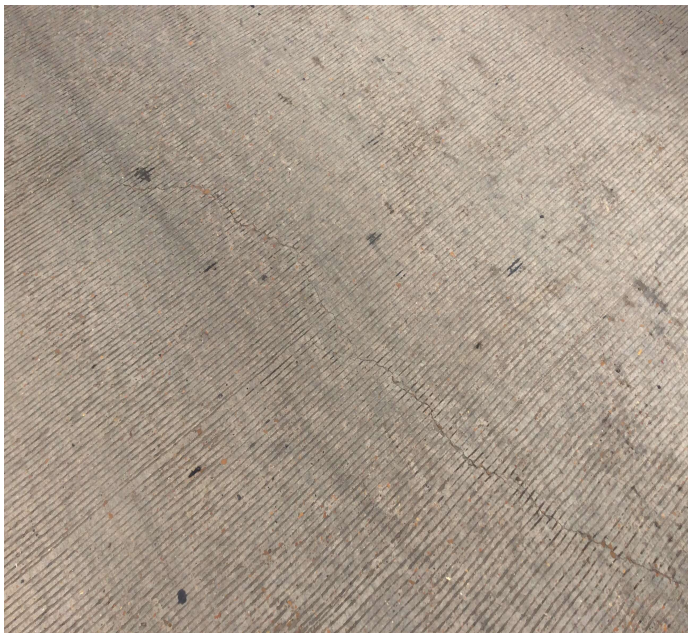
PHOTO 1 Description Typical longitudinal cracks abutment #2 approach slab spaced 6'+-
