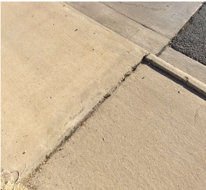
PHOTO 1 Description Abutment #2 right sidewalk has settled 1" at bridge end.
